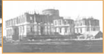
Capitol under construction—1860-74
